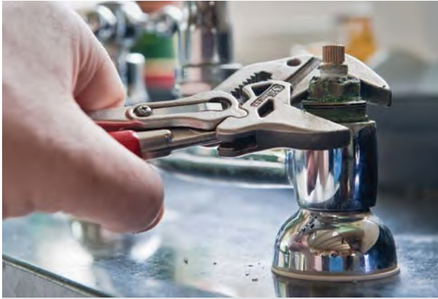
Fix leaky faucets. One drip per second wastes 1,661 gallons of water and can cost you up to $35 per year.
